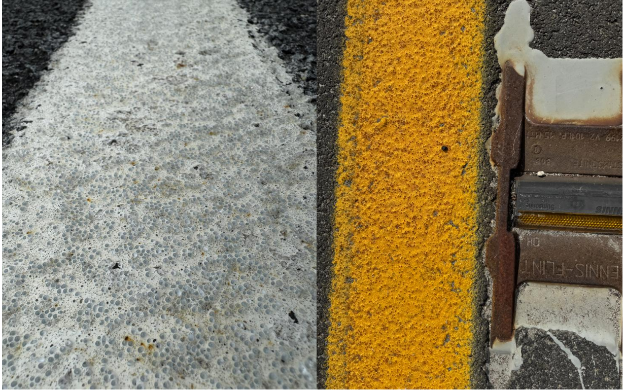
Figure 22. Images of Markings in Good Condition.
