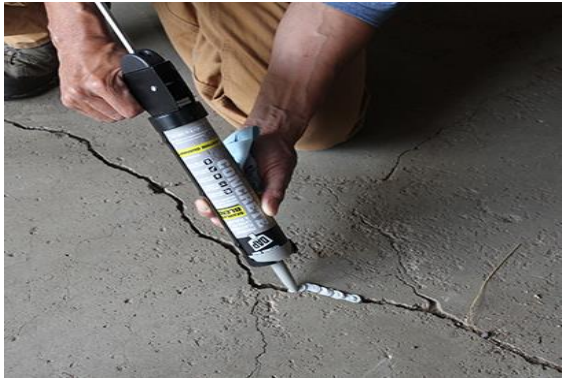
Preventive maintenance like seal joints and cracks
