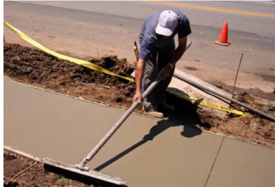
Essential maintenance like repairing or replacement of damaged parts
